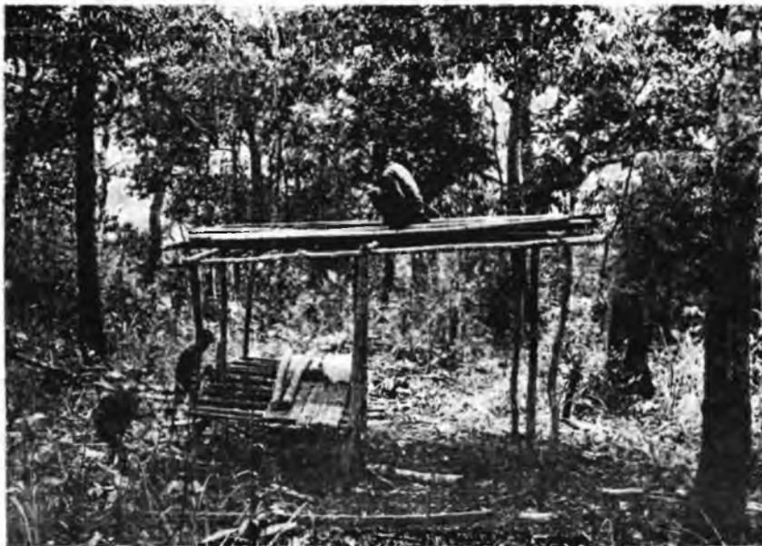
Fig. 1. Building a merit shelter stretching over pathway leading to the village.
