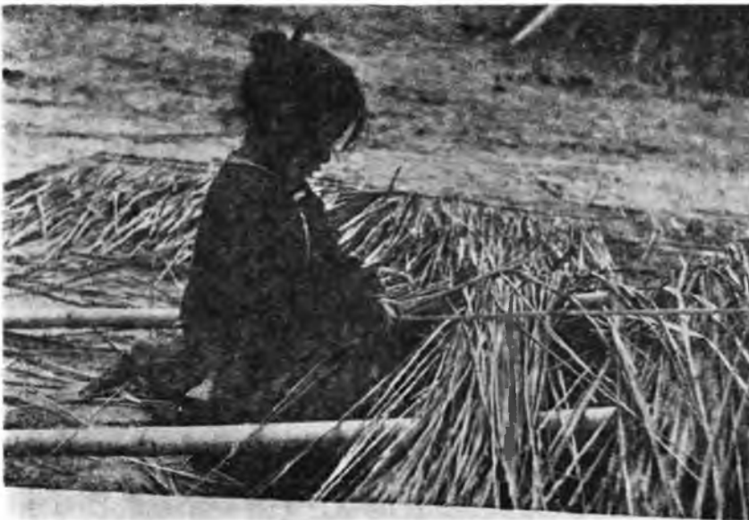
Fig. 2. A Kammu girl weaving cogongrass into building material.
