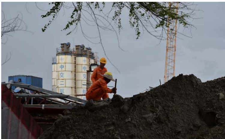
Figure 8. Foreign labor at work on the construction of the Sinamale' Bridge. Photograph by R. Michael Feener.
