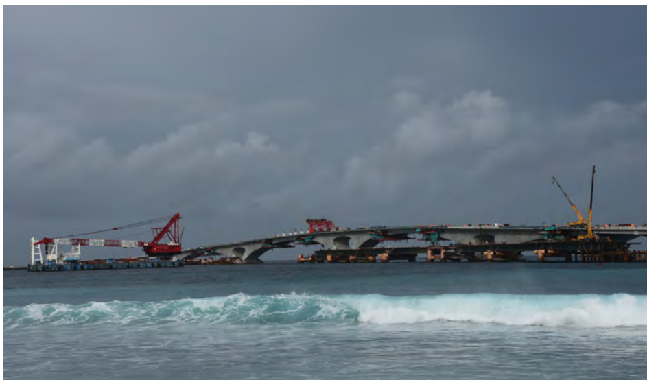
Figure 2. Construction work on the China-Maldives Friendship Bridge. Photograph by R. Michael Feener.
